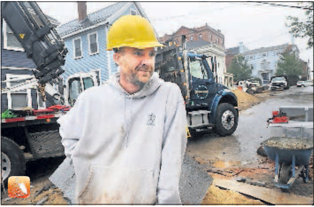
Charlie Anderson, Lead Mason for Piscataqua Landscaping, talks about how important and special it is to be a part of creating the African Burying Ground Memorial Park in Portsmouth. They hope to have the project completed by Thanksgiving. PHOTO BY DEB CRAM/SEACOASTONLINE.COM
